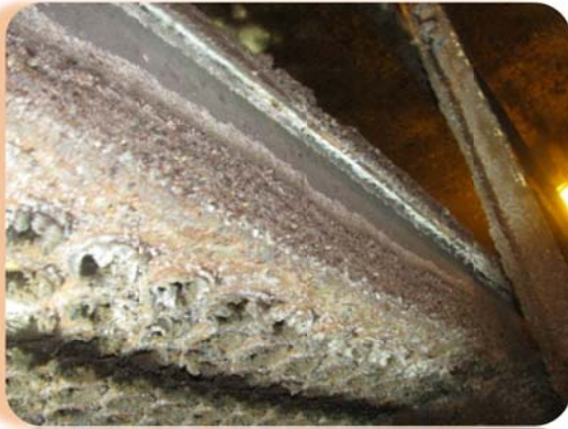
Catwalk Corrosion
