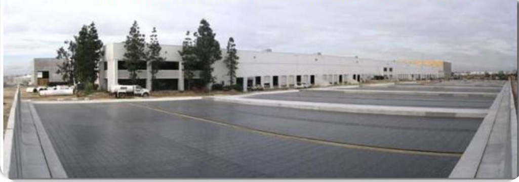
Biofilter at Inland Empire Regional Composting Facility Prior to Media Placement
