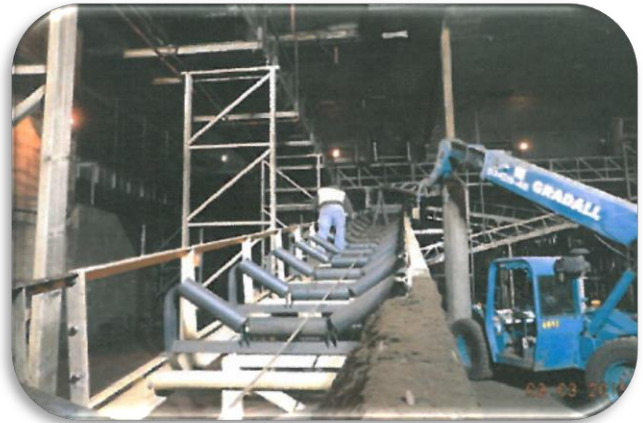
Belt Conveyors #18 Modifications
