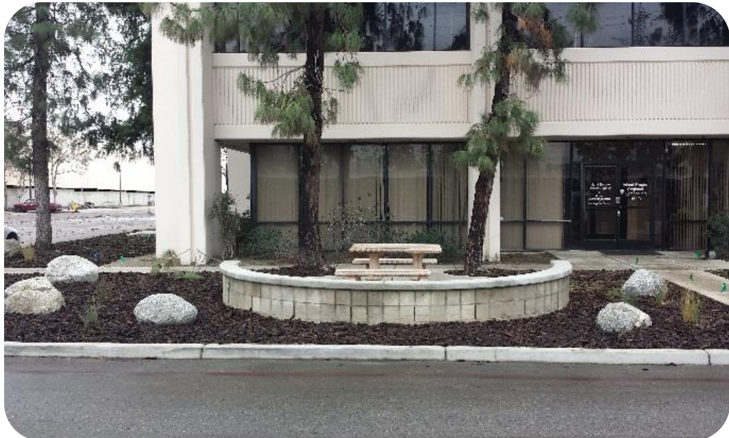
Operations patio area
