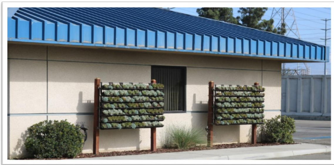
Scale house with living wall
