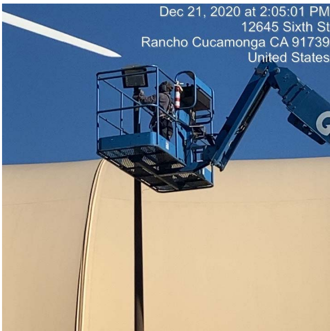
Staff repairing an outdoor light
