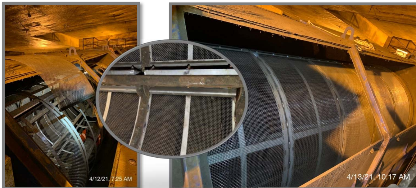
WSM Trommel Screen Tensioning Upgrade
