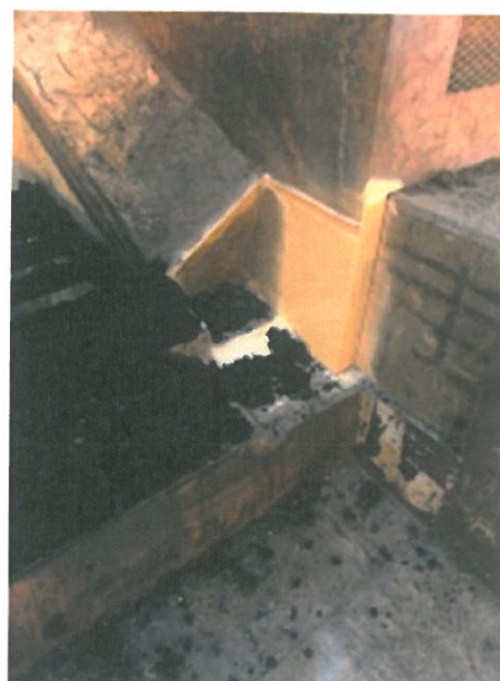
Biosolids hopper after repair
