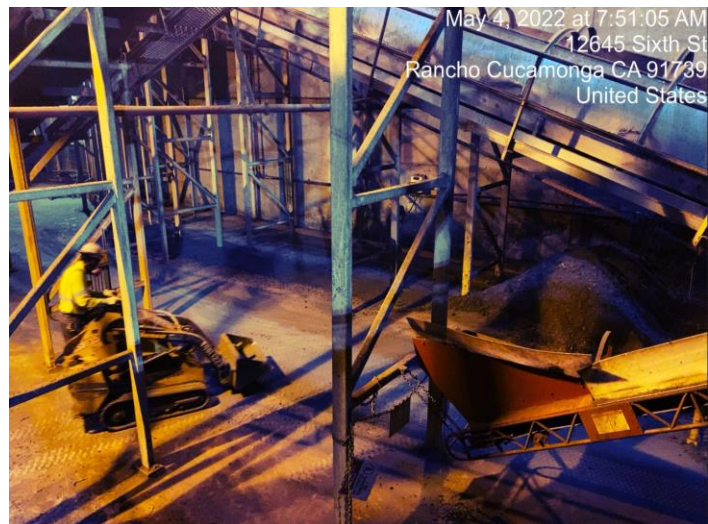
Housekeeping in the basement
