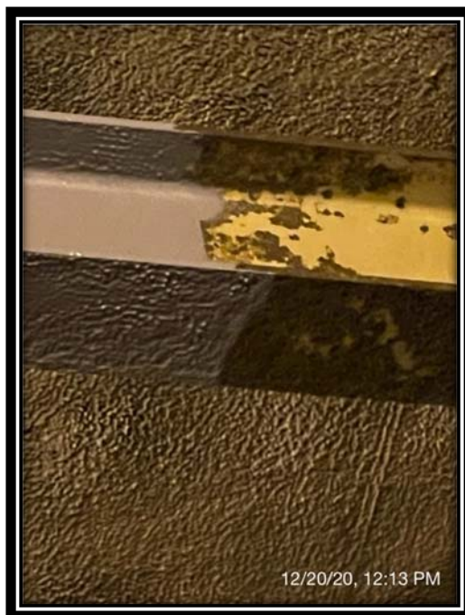
Belzona 1111 "Super Metal" application to main conveyor support I beam.
