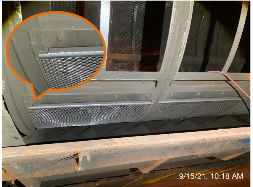
Repaired screen cloth with IERCA designed improvements
