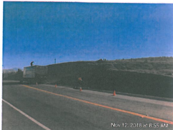
SoilPro applied to a hillside for erosion control via blower truck.
