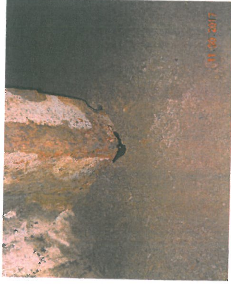
Corroded Column
