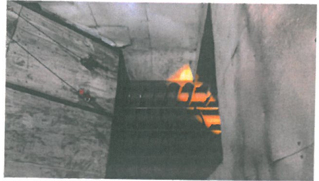
Installing Chute / Job Complete
