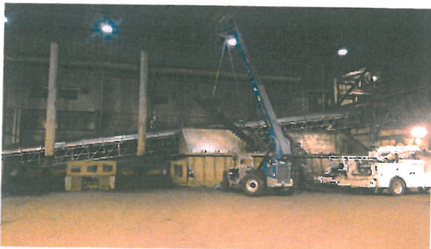
Removing Old Augers
