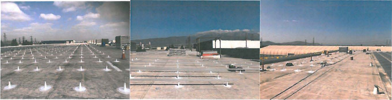
Solar panel construction on the IERCF roof
