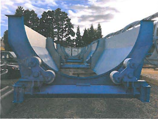
New Trommel Construction
