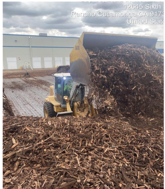
Installing biofilter media
