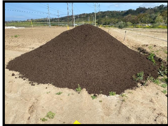
Compost being Applied at DOT Jobsite
