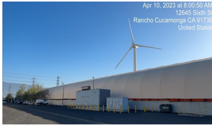
IERCF Compost Storage Facility
