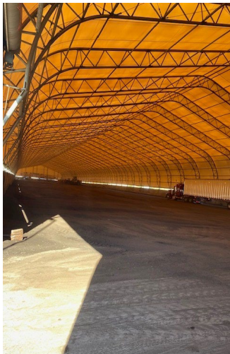
Storage Tent Empty
