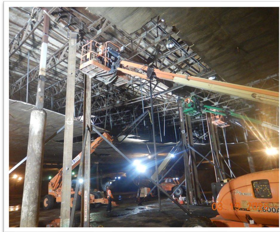
Structural Repairs in Progress
