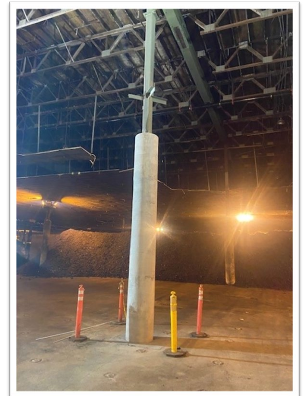
Column After Repair
