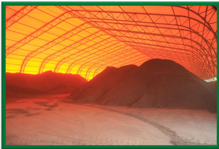
Compost Storage Facility
