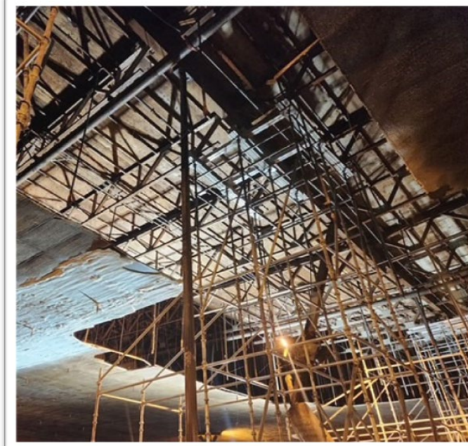
Scaffolding and Shoring Installation
