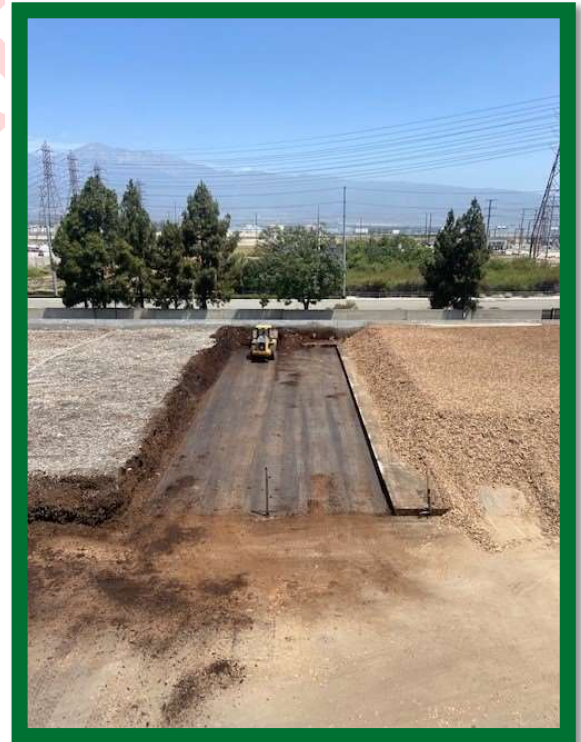
Biofilter Replacement
