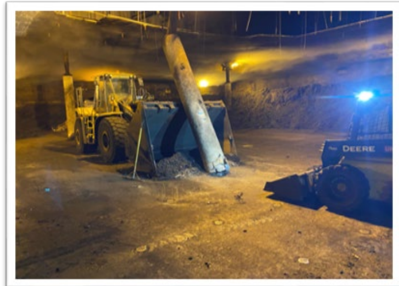
Loader Reinforcing Column
