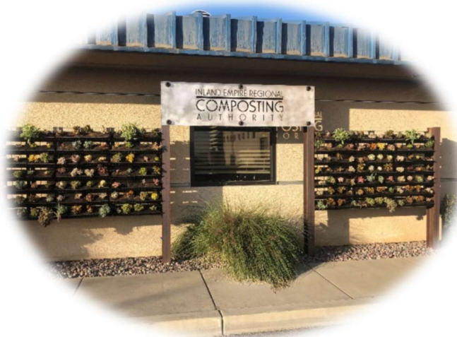
Living Wall at IERCA Headquarters
