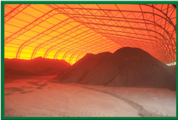
Compost Storage Facility
